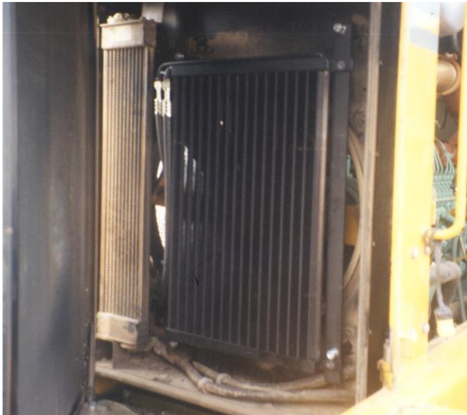
Condenser mounted in position.
